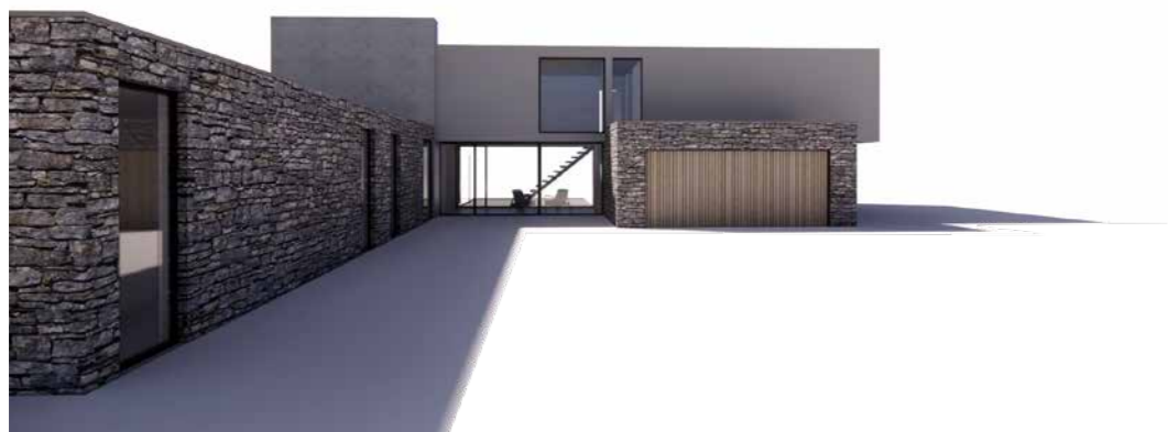
External View (North East)
